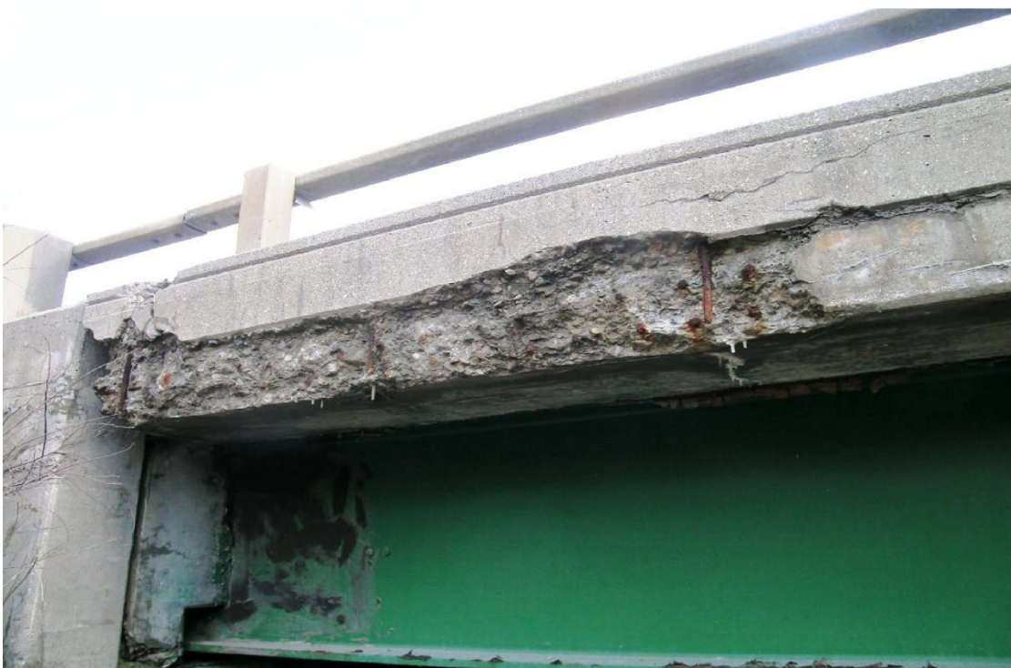
Fascia Deterioration
