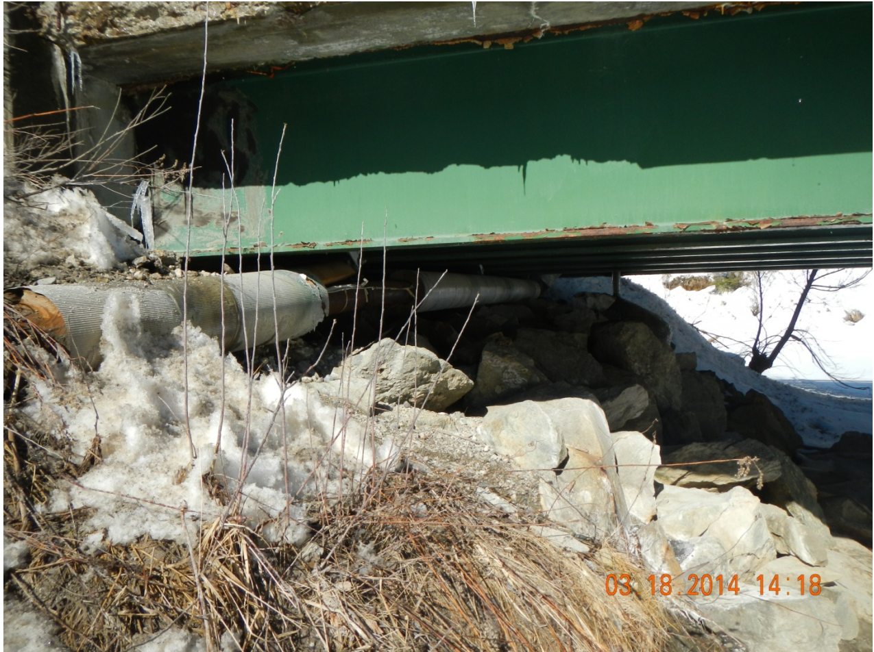
Figure 3. Utility Conduit below Northwest end of Bridge
