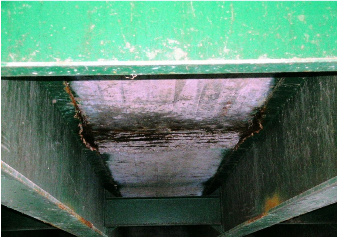
Deck Deterioration
